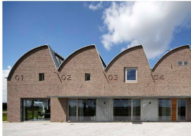
Soft curved Zig Zag Roof and Numbering
